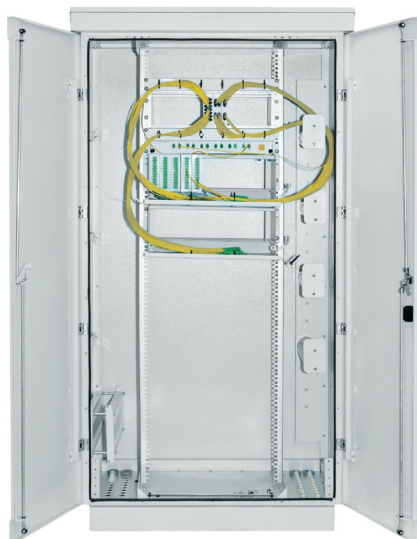
Street Cabinet PU-10 with FTTX equipment
